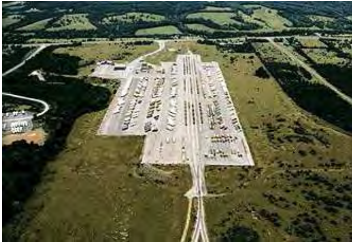
Figure 3.1 Aerial View of Virginia Inland Port
